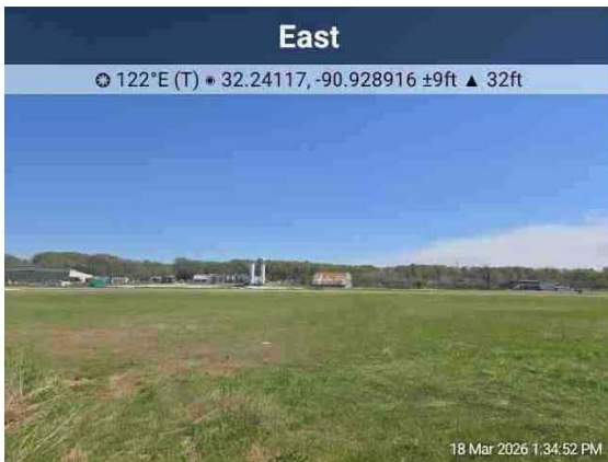
29. Typical view of site
