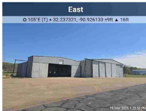
6. View of Hanger B2/B3
