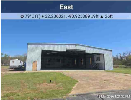
7. View of Hanger B4
