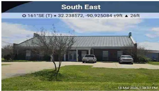
33. View of fire station
