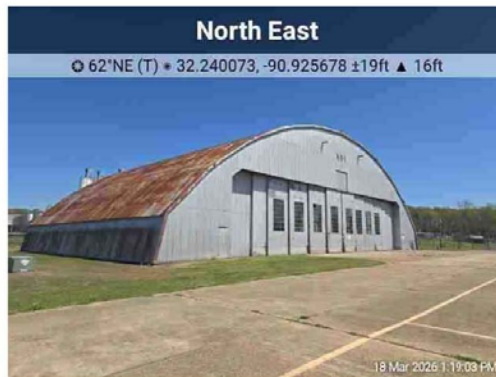
4. View of Hanger B1
