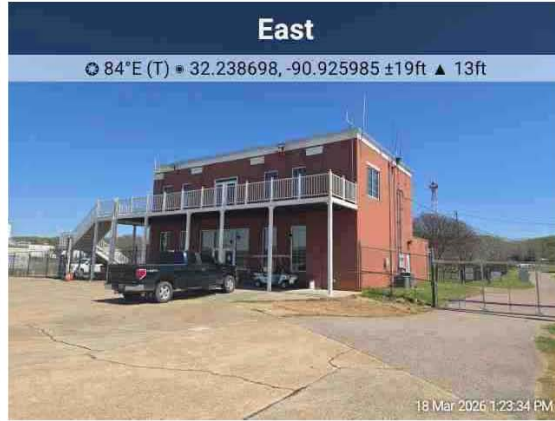
8. View of Terminal/Office
