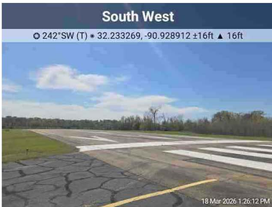
11. Typical view of site - runway
