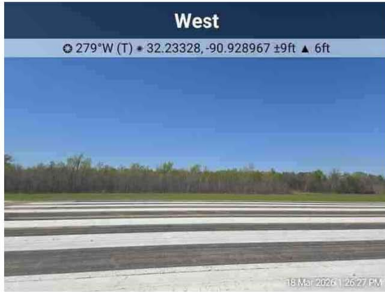
13. Typical view of site - runway
