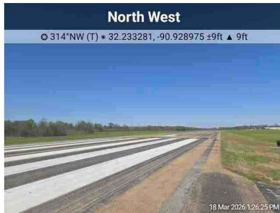
12. Typical view of site - runway
